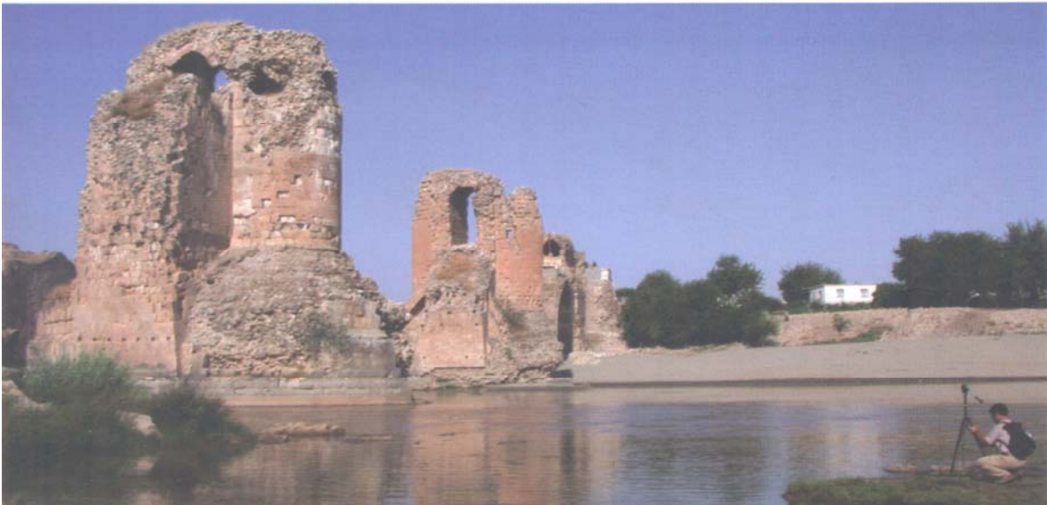
Photo of the bridge
