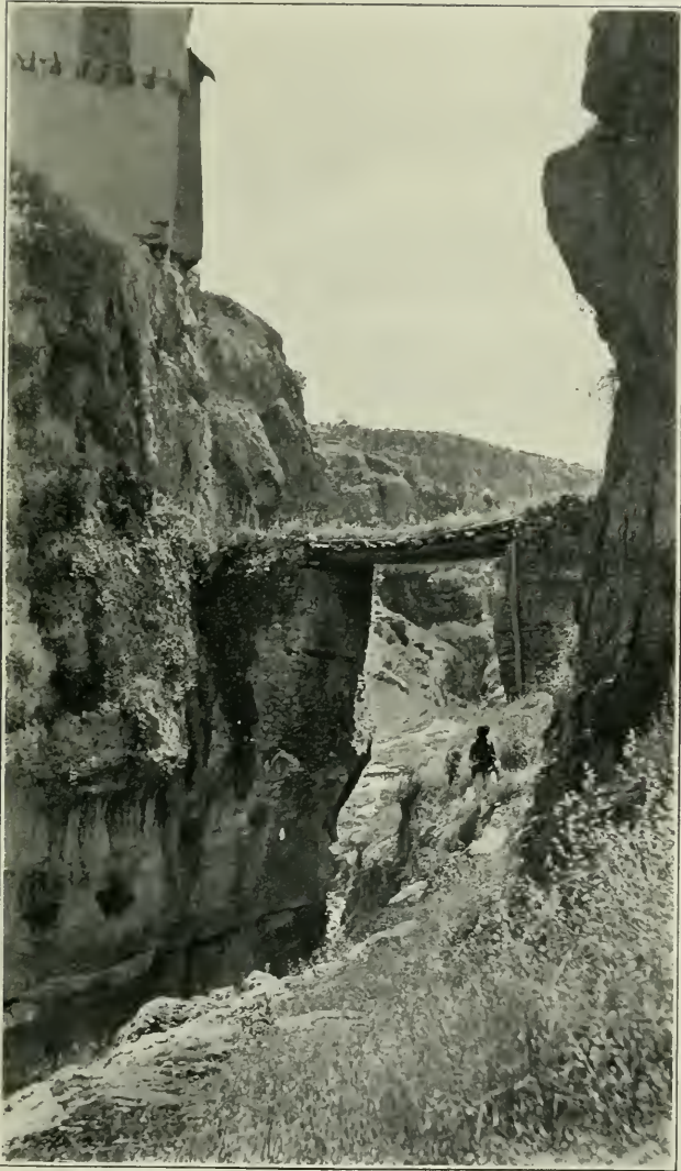
THE ONLY ROAD TO RAWANDUZ FROM THE NORTH.
