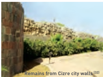
Remains from Cizre city walls (32)
