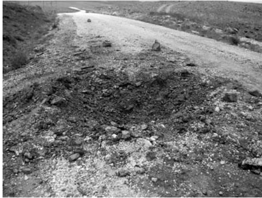
Landmine damage on the way to Taşnacak, July 2006
