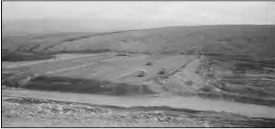
Figure (37) Spill way in kurdistan region
