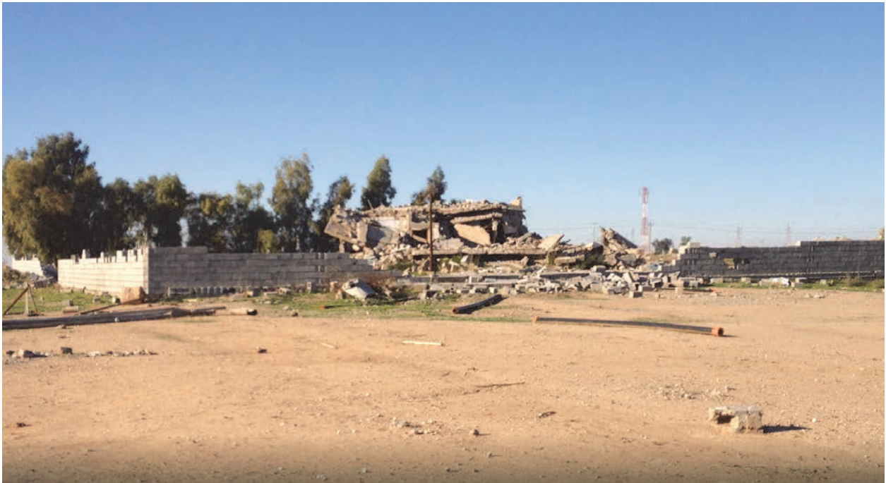
One of two houses in Idris Khaz'al hit by an airstrike, with collapsed roof. ©2015 Human Rights Watch
