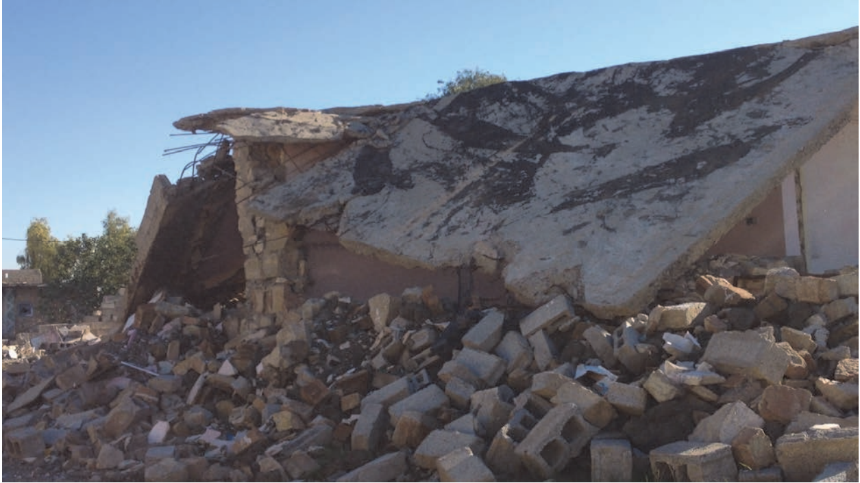
Houses destroyed by bulldozers in Idris Khaz'al after February 1, 2015 © 2015 Human Rights Watch
