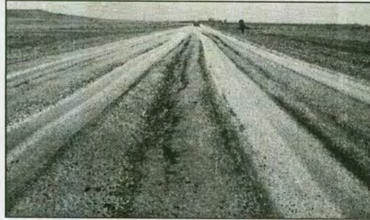
Figure (2-1) Rutting Phenomena (Qetewy-Dustepa Road Erbil Governorate/2011)
