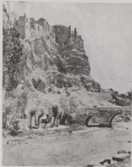
(a) BRIDGE AND CASTLE AT KHOSHĀB (p. 155)
