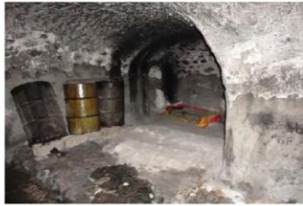
(1) - View into room 2.09
