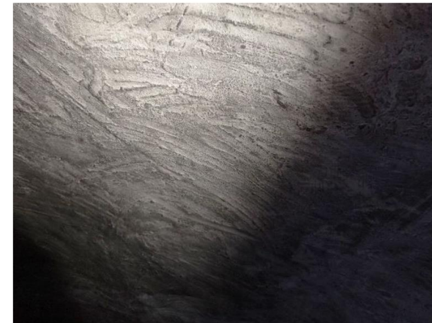
Above left , Oil Hall 3, area of historic lime plaster showing beneath a modern cement screed
