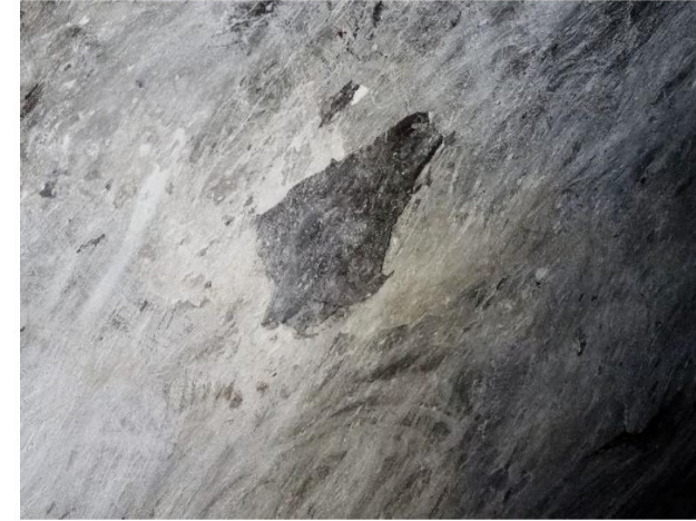
Above left , Oil Hall 3, area of historic lime plaster showing beneath a modern cement screed
