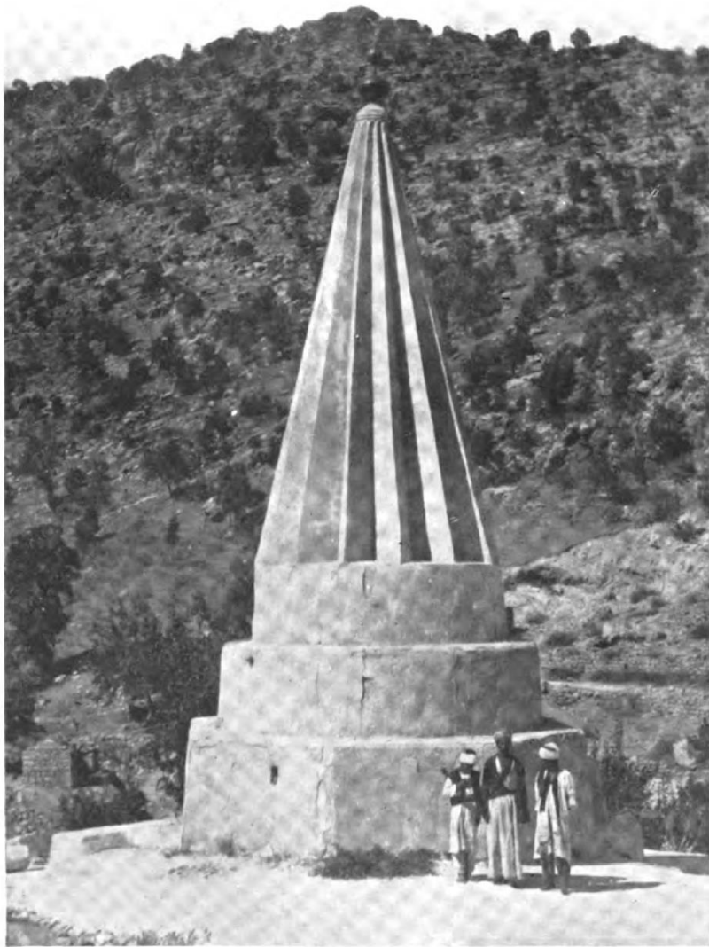
THE ROOF OF SHEIKH SHEMS-ED-DIN AT SHEIKH ADI. Round this spire the sacrificial bull is driven. (See page 203.)
