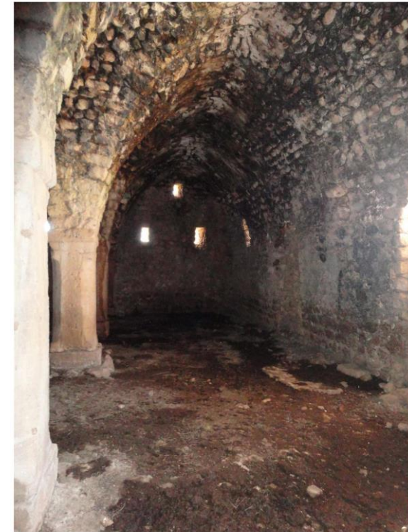
Khaana Ezid interior, 2011 – In the northern part of the building there is a two-span hall, similar to the chambers of the Yazidi temple complex. The vaults rest on lime stone centre piers.
