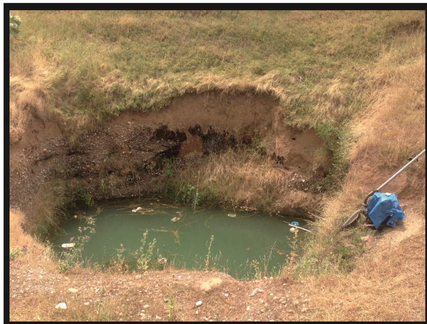
Plate 3.1: Large diameter well (6mx8mx8m) near to Grdanaze village (South of Saidsadiq District)
