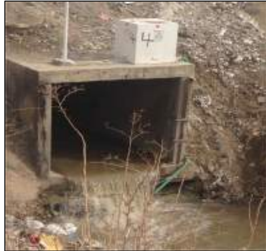
Fig.(1.3): Sewer Box Outlet in Gwmdi Kanaswra, (Researcher)
