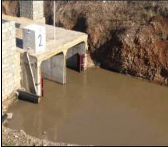
Fig.(1.2): Double Sewer Box Outlet in Awabara Sub- District, (Researcher)
