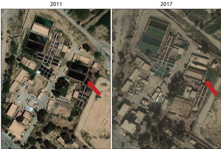
Figure 3.12 Drinking Water Treatment Plant in Al-Jorah District of Deir ez-Zor City, 2011 and 2017
