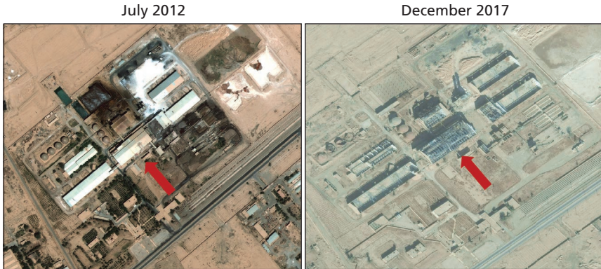
Figure 3.2 Damage to Sugar Factory in Industrial Zone on N-7 National Highway, Eastern Side of Euphrates Near Deir ez-Zor City
