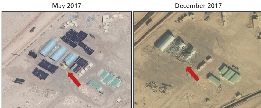
Figure 3.3 Damage to Storage Facility Near Kahara Air Base in Abu Hamam
