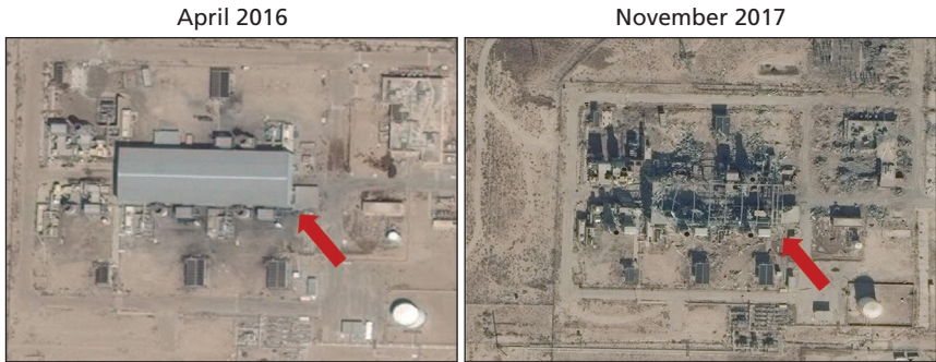
Figure 3.10 Damage to Thermal Natural Gas Power Plant, Omar Oil Field
