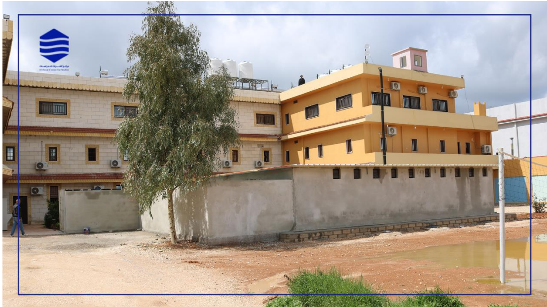
Building of Orkish Center for Rehabilitating Children from ISIS families.
