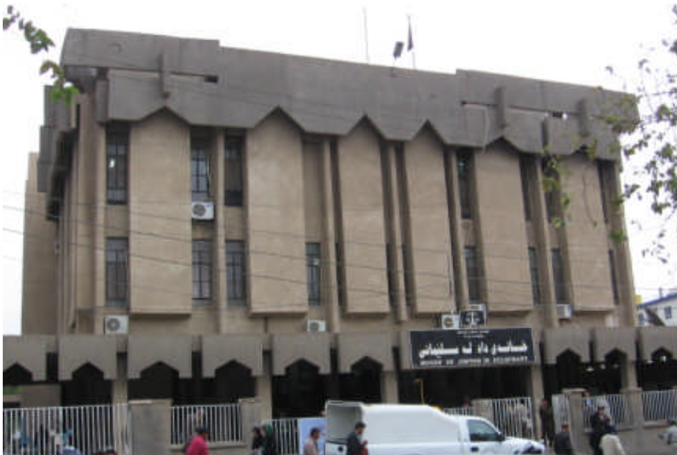
Sulaymaniyah House of Justice 2008 (a new court house is under construction) (photo by author).
