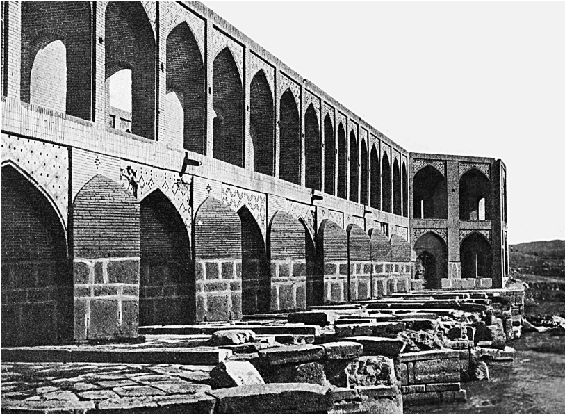
Khaju Bridge, Isfahan, ca. 1911
