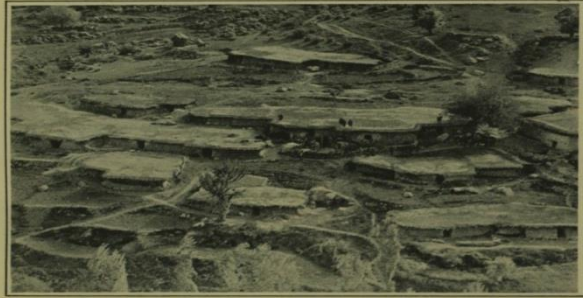
A TYPICAL VILLAGE IN THE DISTURBED AREA OF KURDISTAN, WITH ROUGH STONE HOUSES HAVING FLAT ROOFS OF MUD AND BRUSHWOOD: AN AIR PHOTOGRAPH ENTITLED "ARMY PATROL ENTERING HAFNADAKA."
