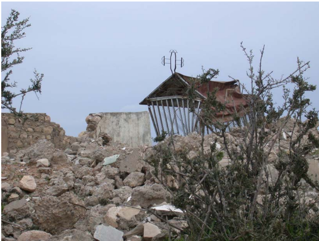
Figure 74 Rubble of a church in Bakhitme. All three churches of the village were destroyed during 1987.
