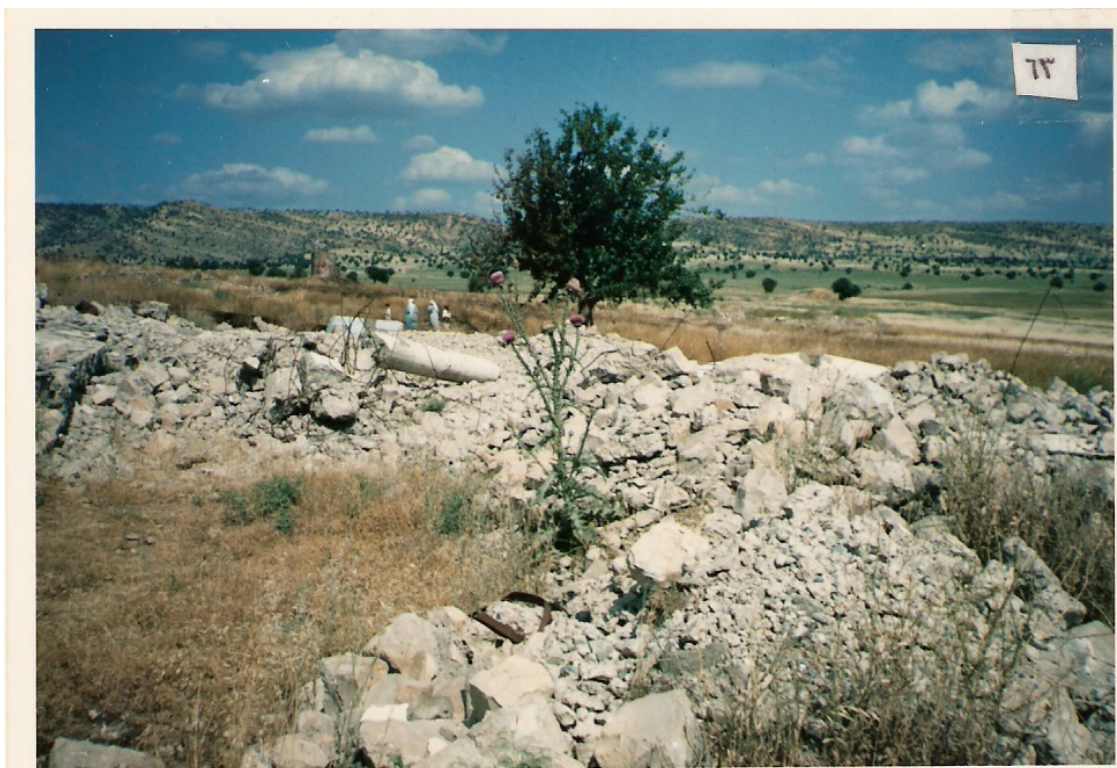
Figure 71 Rubble left from the destruction of Mar Abraham church in Levo, Zakho region destroyed 1988. Photo courtesy of the Nineveh Center for Research and Development, Qaraqosh, Iraq.
