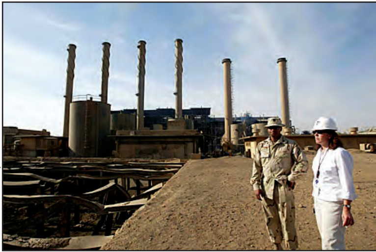
Figure 96. Contractor Janene Van Deroef and Captain Rodrick Pittman of the 40th Engineering Battalion make a site inspection at the Baghdad South power plant.
