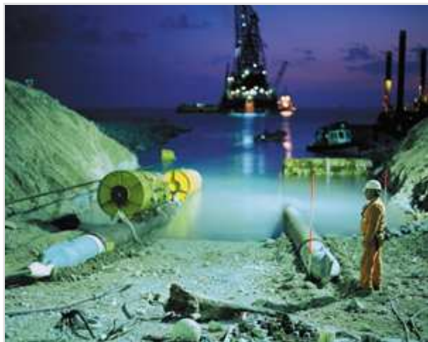
Construction of South Stream pipeline (c) South-stream.info
