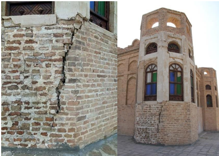
Fig. 6.b–g: The severe damage to the attic seen after the earthquake on November 12, 2017. (Photo by Nawzad Latif, Archive of the Directorate of Antiquities of Garmian).
