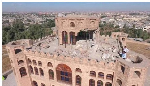
Fig. 6.b–g: The severe damage to the attic seen after the earthquake on November 12, 2017. (Photo by Nawzad Latif, Archive of the Directorate of Antiquities of Garmian).
