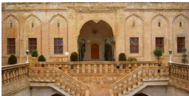
Fig. 8 Facade of Mardin PTT House
