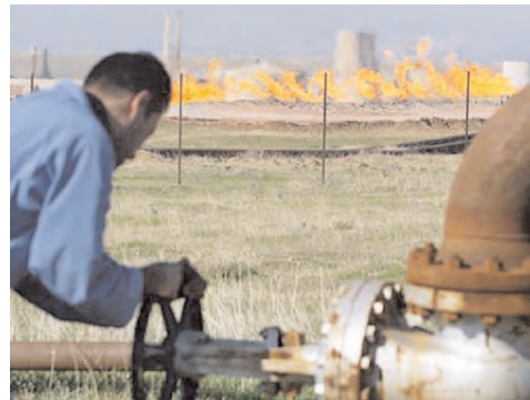
An oil worker tending to a supply pipeline in Iraqi Kurdistan.
