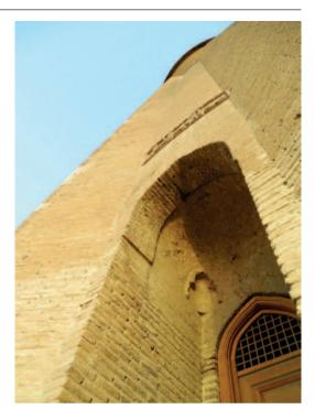
Figure 6. Arched entrance of the tower of Gonbad-e Kāvus with one of the two stucco niches
